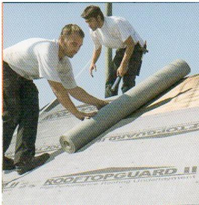
**SITE PROTECTION:** Prior to loading the roofing materials onto the RoofTopGuard product, it is recommended that a roof jack, with planks, toe boards, or a strong platform be secured to the underlying roofing deck to prevent slippage of stored materials on steep sloped roofs (greater than 4 : 12 pitch). See OSHA regulations (Standard 29 CFR), fall protection systems criteria and practices – 1926.502.
